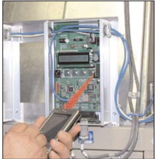
Figure 25. EB-Link Communication Detail
